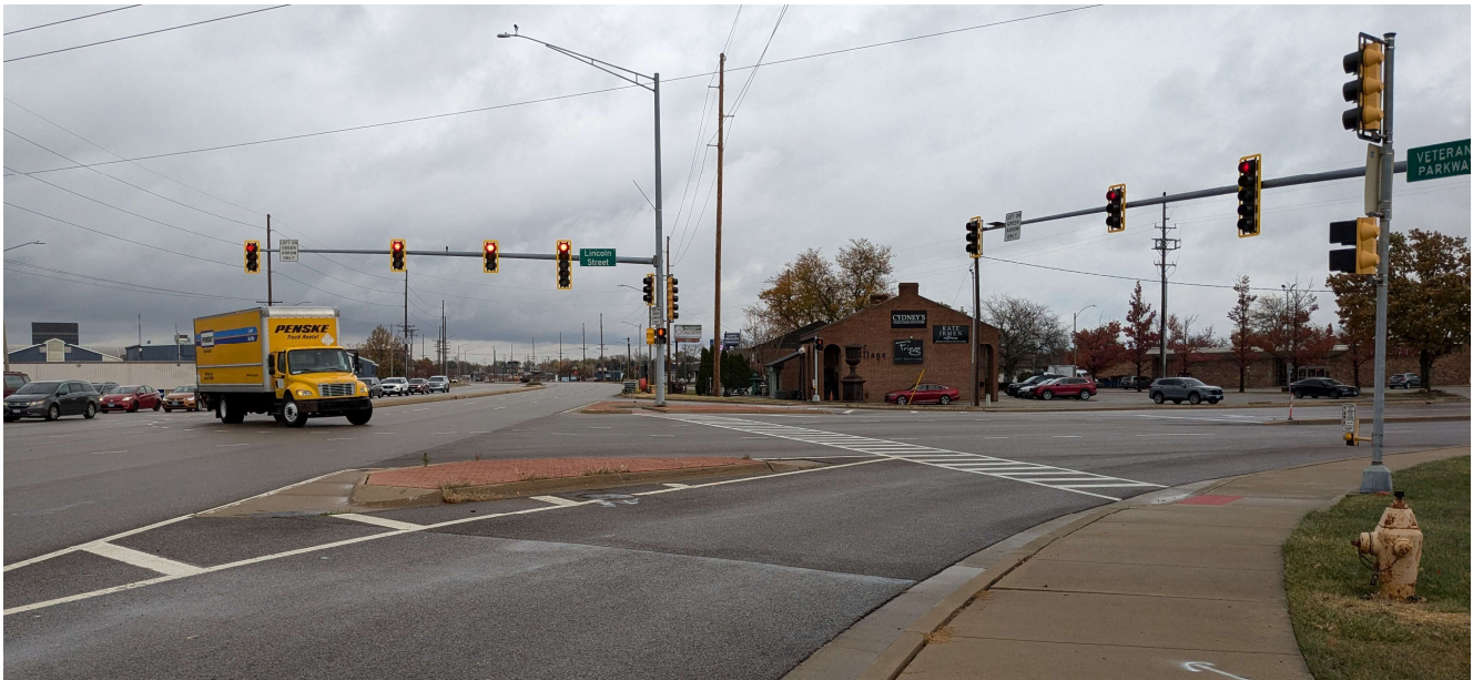
Large corner radii allow vehicles to make right turns at higher speeds.
