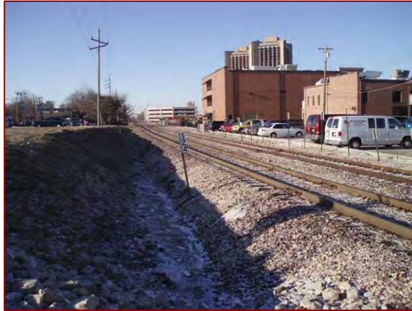
Figure 22. The Union Pacific Railroad represents a barrier to bicyclists and pedestrians
