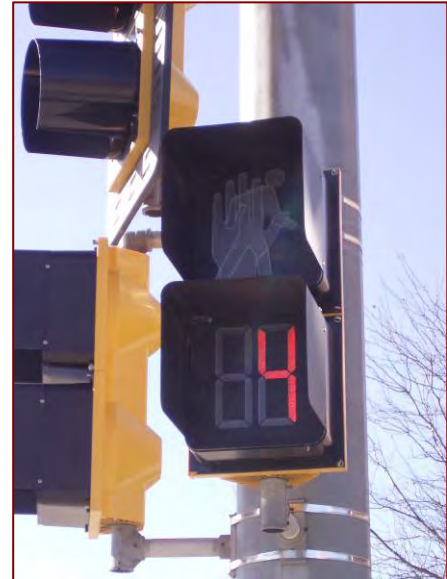
Figure 21. Pedestrian countdown signal at the intersection of College Avenue at University Street
