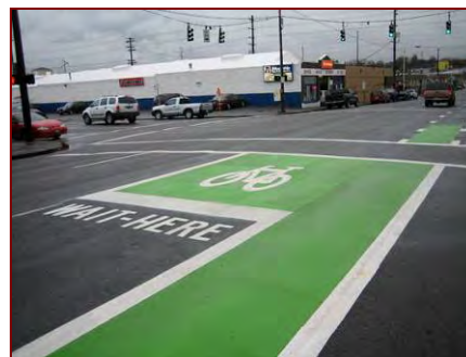
Bike boxes have been installed at several intersections in Portland, OR where right-turning motorists conflict with through bicyclists
