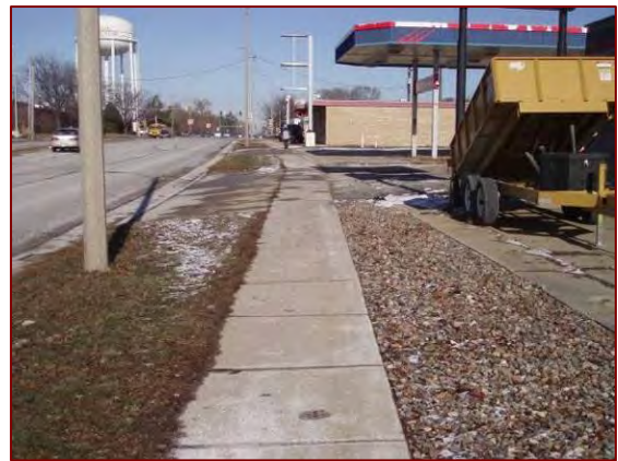
Figure 2. Portions of Main Street north of College Avenue have four-foot wide sidewalks
