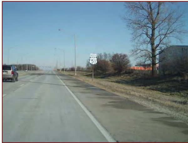
Figure 11. Eight-foot wide shoulders exist on Main Street near Interstate 55, which could accommodate bicycle travel
