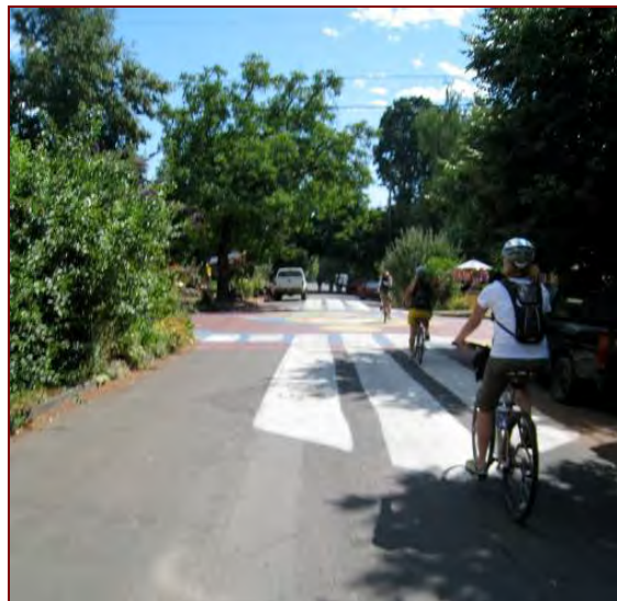
Example of patterned pavement used for traffic calming purposes
