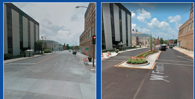
One example of a successful road diet implementation on Front St. in Bloomington
